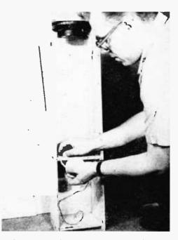
AFTER wiring the speakers, seams of upper chamber are sealed with Mortite house putty.
